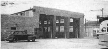
This new maintenance garage, last step in an $8,000,000 modernization program in Columbus, O., was . . .
